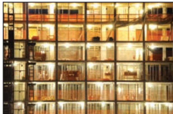
One application for Temporary Lighting
