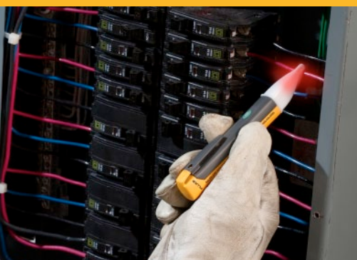
1AC-II with beeper, on-off and self test
