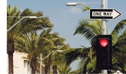
traffic signal controls
