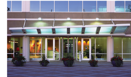
outdoor facility lighting
