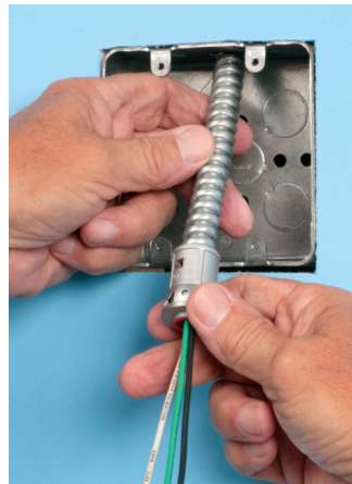
Snap fitting onto cable.
