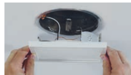
Friction clips for recessed housings
