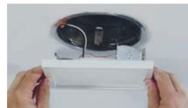
Friction clips for recessed housings
