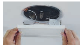
Friction clips for recessed housings
