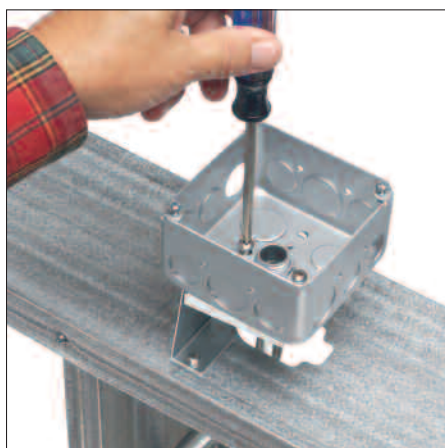
6 Attach 4x4 metal box to the stand-off bracket with screws (not provided) through pre-drilled holes in bracket.
