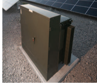
Medium voltage step-up transformer
