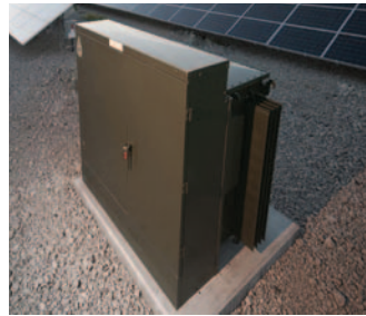
Medium voltage step-up transformer
