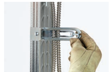
Once cables are inserted, wrap zip-tie around the end of the support to secure the cables
