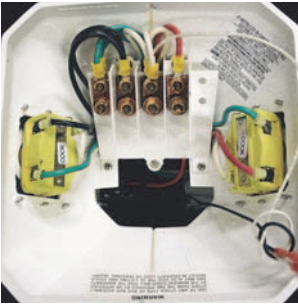
Copper Busbar with Ratings up to 140 A
