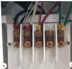
Copper Busbar with Ratings from 250 to 500 A
