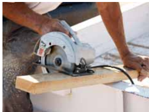
Construction Site Application
