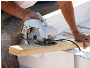
Construction Site Application
