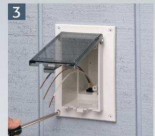
3 Attach IN BOX with stainless steel screws (provided).
