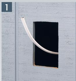
1 Cut a 3-1/4" x 5-1/2" hole in substrate. Pull wiring.
