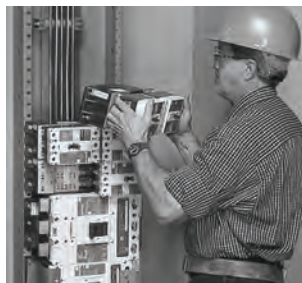
Panelboard Installation
