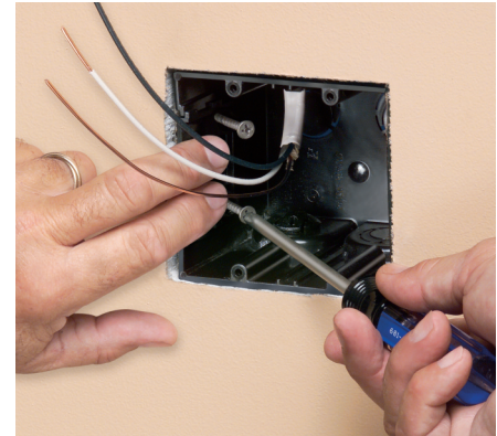
3 Mount ONE-BOX directly to stud with shipped in place screws.
