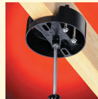
1 Convenient. Gripping tangs hold box in place temporarily, until the center screw is tightened.
