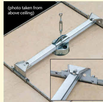
2 Place box over hole. Place ends of support bar over the ceiling grid (tees).
