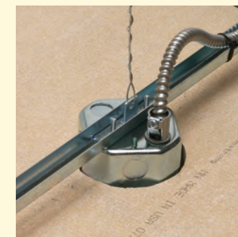
4 Cable pulled through cable connector (not supplied).
