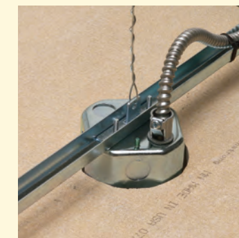
4 Cable pulled through cable connector (not supplied).
