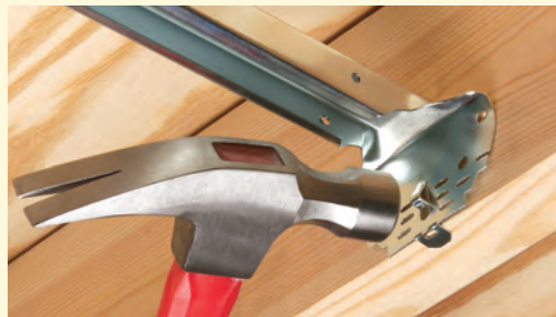
1 "Tooth" holds bracket temporarily in place.
