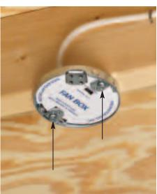
4 Replace the mud cover. Remove the #10 screws indicated above...
