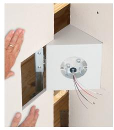
3 Cut and position drywall to fit around the box. (Note captive screws in box). Install fan or fixture per manufacturer's instructions using captive installation screws.
