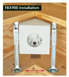
1 For proper fan/fixture installation, use supplied template to level and position brackets between rafters. Remove captive screws on sides of brackets and use to attach FBX900 assembly to rafters.
