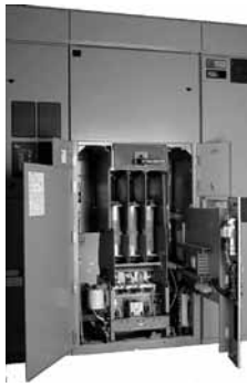
50L7 Vacuum Retrofit
