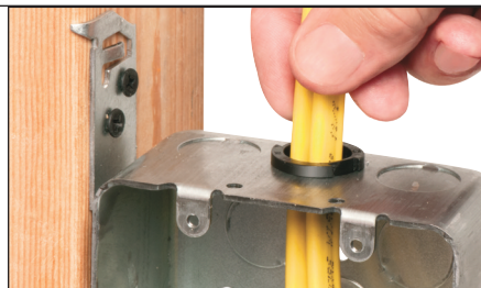
2 Insert cable(s) into individual openings.
