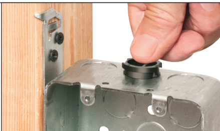
1 Push connector into KO with light finger pressure.
