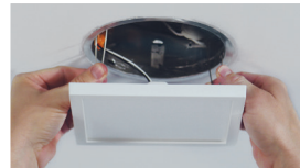
Torsion springs for recessed housings
