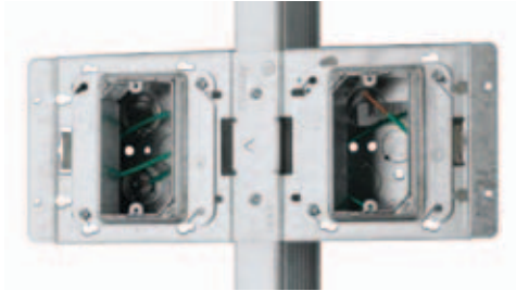
Power on both sides of the stud
